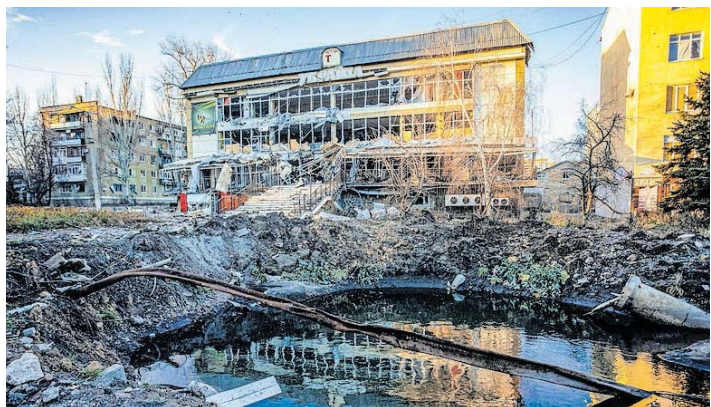
A destroyed building in Bakhmut, Donetsk region, amid the Russian invasion of Ukraine on November 29. Once known for its vineyards and cavernous salt mines, Bakhmut has now been dubbed "the meat grinder" due to the brutal trench warfare, artillery duels and frontal assaults that have defined the brutal fight for the city for over six months. PHOTO | AFP
